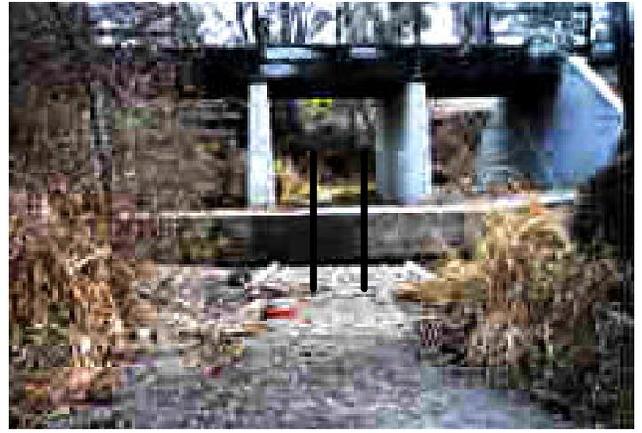
Photo #1. Drop structure (three foot) on Arroyo Mocho at Stanley and Murrieta Blvds at the old Southern Pacific railroad bridge in Livermore. A slot as shown needs to be cut in the concrete to allow fish passage.
