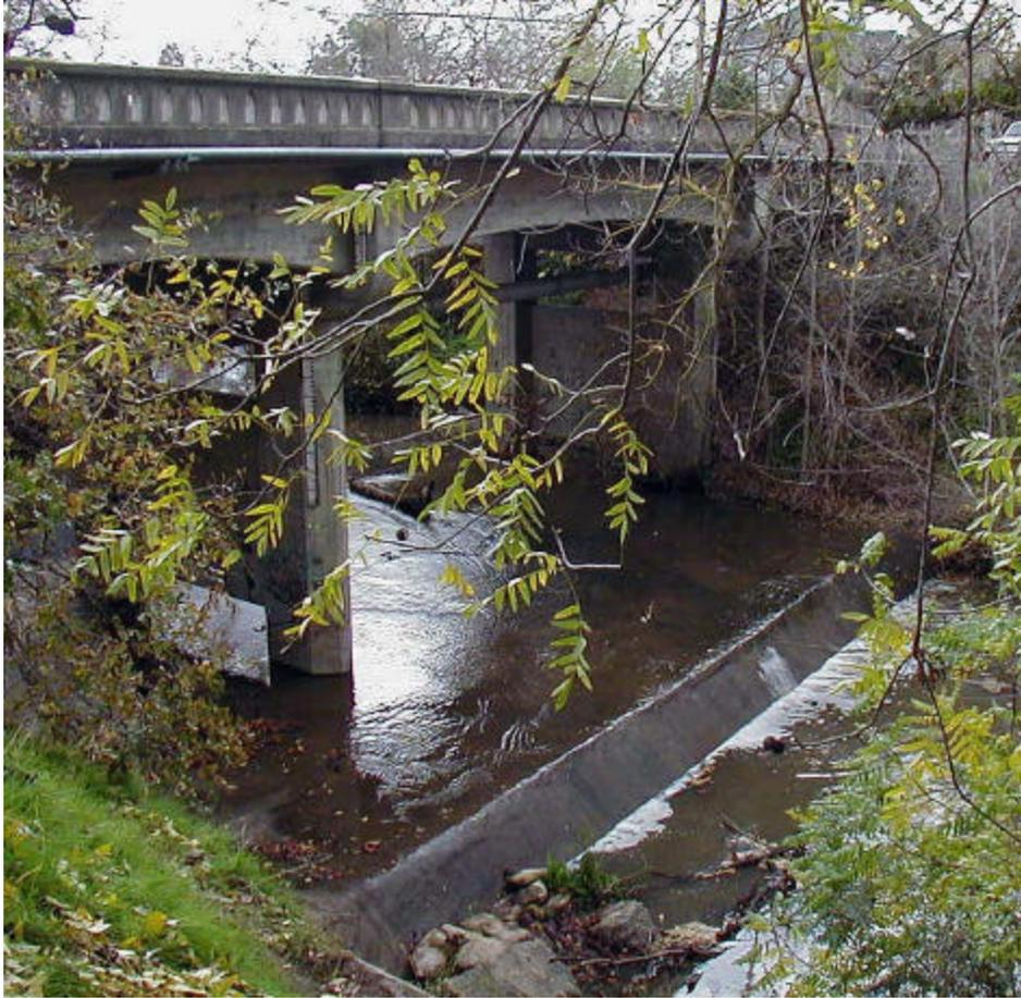
Photo #5. Drop structure (a few feet) on Arroyo Del Valle where Division Street crosses in Pleasanton. At low to moderate flows this structure blocks fish passage due to the flat apron above the drop.
